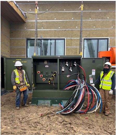
Fergus Electric Cooperative Linemen Mark Schwomeyer and Dakota Wahl prepare to connect the service wires to the transformer. | PHOTO BY LOUIE HOULD
