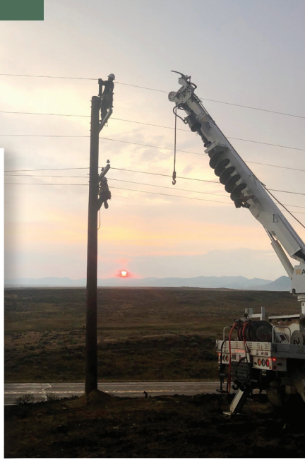
Fergus Electric Cooperative Linemen tie in a conductor on a freshly set pole between Bohemian Corner and Grass Range in February. | PHOTO BY LOUIE HOULD
