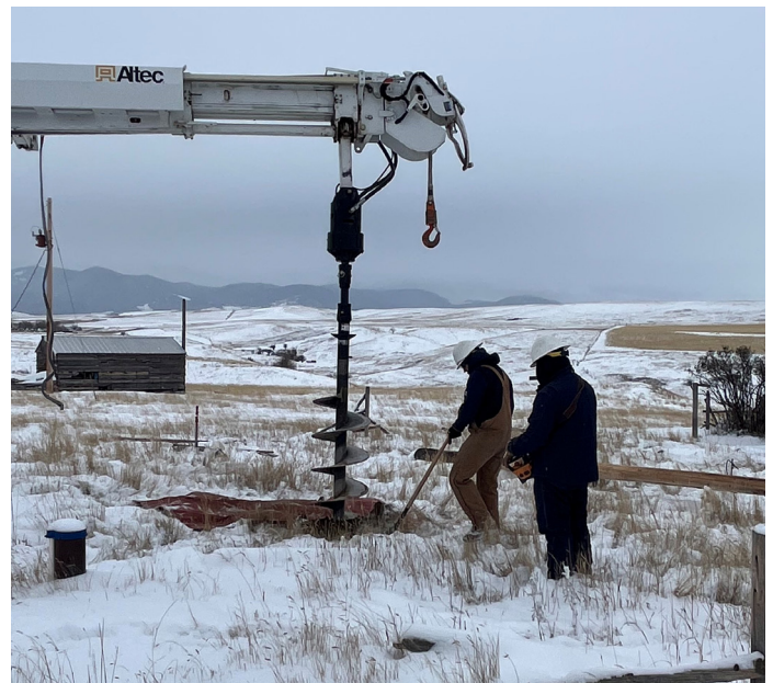
Lineman Darek Dygert and Apprentice Lineman Collin Sullivan use a digger derrick auger to dig a hole for a pole being set east of Hilger. | PHOTO BY FERGUS ELECTRIC FOREMAN LOUIE HOULD
