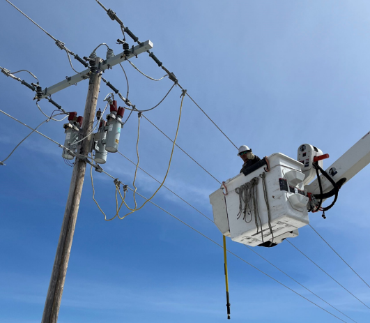
Fergus Electric's Tyson Ruff grounded a power line so crews could work safely. | PHOTO BY LOUIE HOULD
