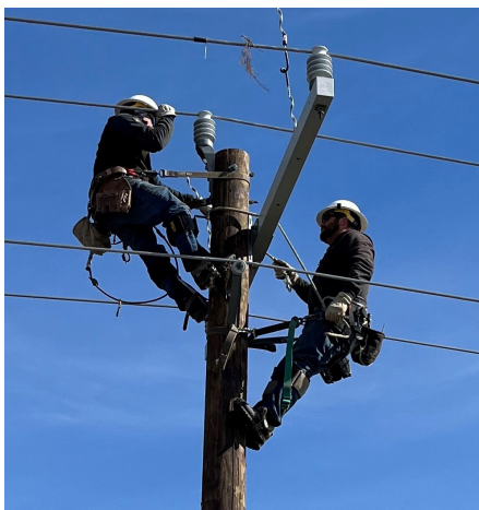
Members of the Fergus Electric crew tie in a conductor on a freshly set pole for Sheridan Electric. | PHOTO BY LOUIE HOULD
