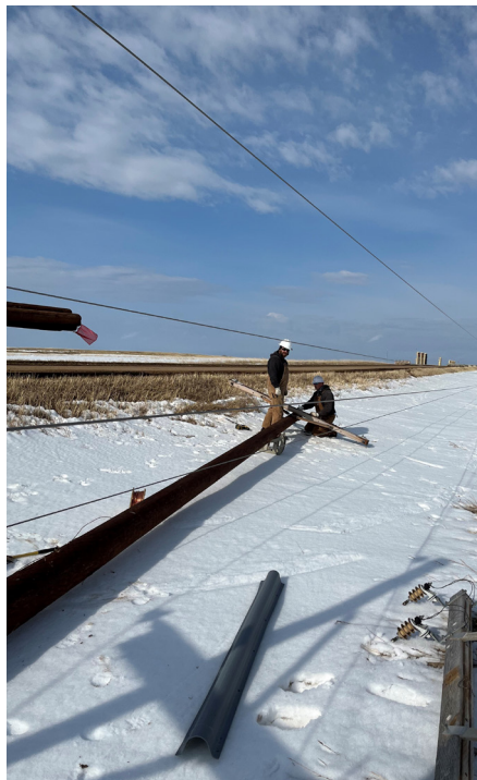
Fergus Electric's Mark Schwomeyer and Tyson Ruff frame a pole after Sheridan Electric suffered major damage during an April storm. | PHOTO BY LOUIE HOULD
