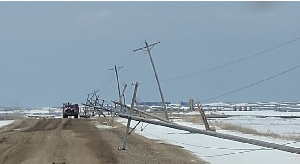
The April storm damage to Sheridan Electric was extensive and widespread, nearly 500 power poles were lost. Fergus Electric sent a five-person team to help. | PHOTO BY MELANIE FORAN
