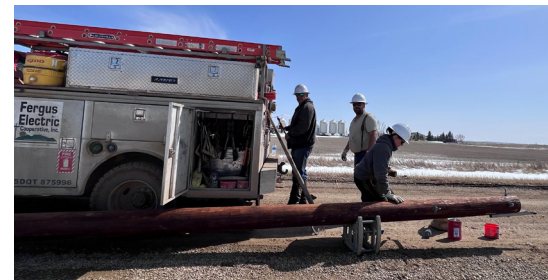
Fergus Electric's Tyson Ruff, Louie Hould and Melanie Foran frame a power pole. | PHOTO BY MARK SCHWOMEYER
