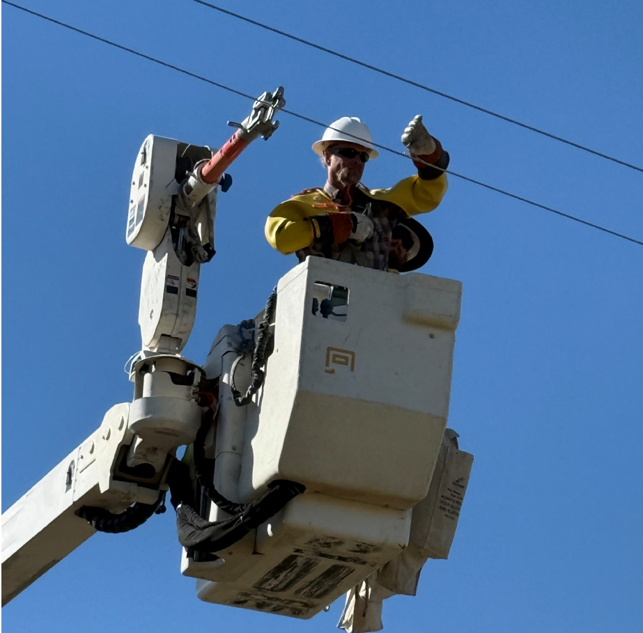
ABOVE: Jason Deffinbaugh repairs a broken conductor strand discovered during one of our drone-assisted line patrols. Deffinbaugh recently was promoted to apprentice lineman. BELOW: Travis Sura is pictured changing out an A1 as part of our pole testing and replacement program. Sura finished the fourth step of seven (hot certification), to becoming a journeyman lineman. | FEC PHOTO
