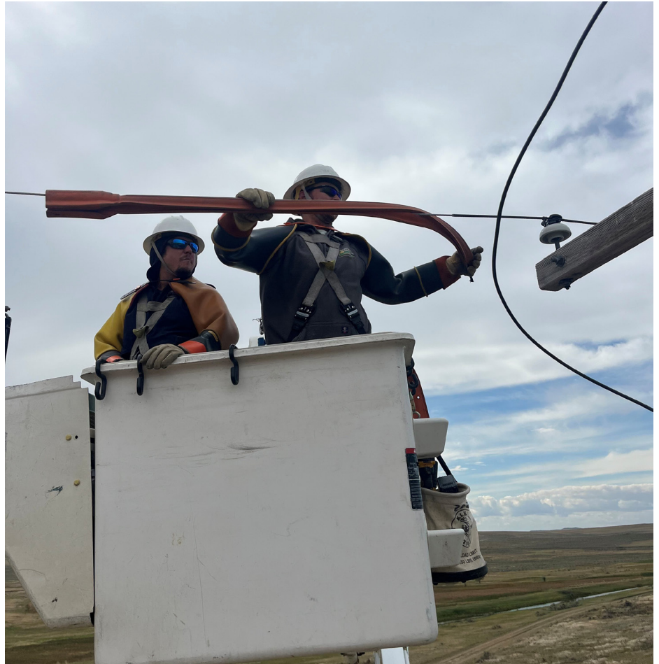
Dylan Rickman safely covers an energized conductor in preparation to hang a sectionalizing device, part of our six-year systemwide effort to upgrade circuit coordination and install new protection equipment. Rickman recently completed his hot certification. | FEC PHOTO
