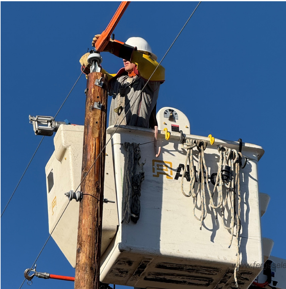
ABOVE: Jason Deffinbaugh repairs a broken conductor strand discovered during one of our drone-assisted line patrols. Deffinbaugh recently was promoted to apprentice lineman. BELOW: Travis Sura is pictured changing out an A1 as part of our pole testing and replacement program. Sura finished the fourth step of seven (hot certification), to becoming a journeyman lineman. | FEC PHOTO
