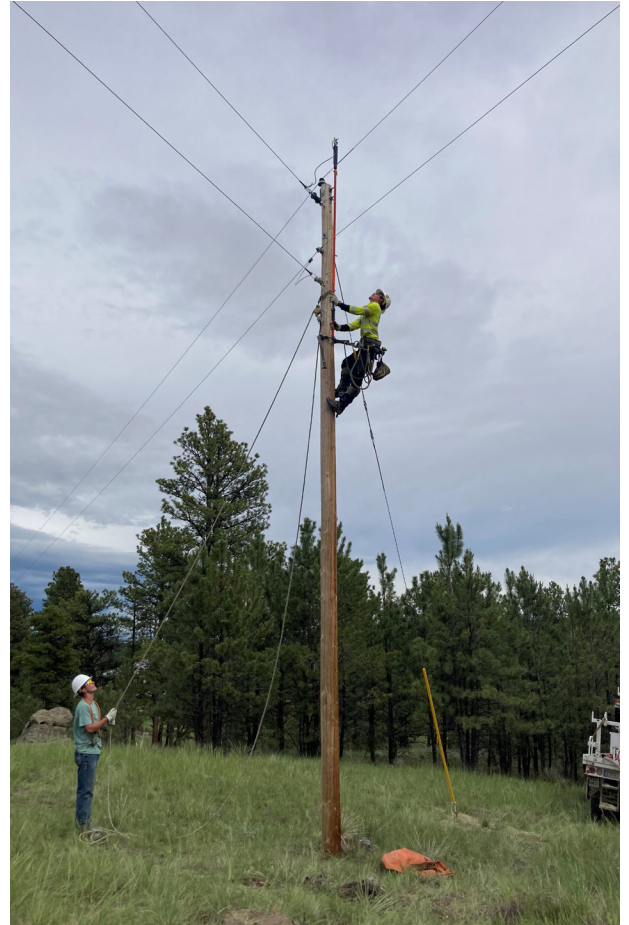
Groundman Dylan Rickman holds a handline while Lineman Andrew Reuterskiold (on pole) removes the ground in preparation for energizing the powerline on a new service in the Roundup area. | FERGUS ELECTRIC PHOTO
