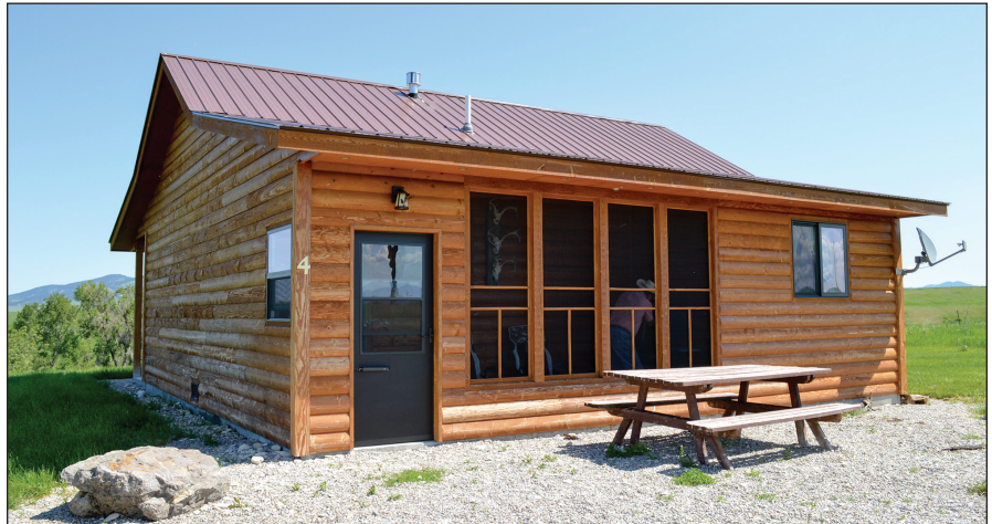
Along with improvements on the original three cabins, a fourth cabin was built in 2016. The cabins are located 10 miles west of Lewistown near Beaver Creek.
