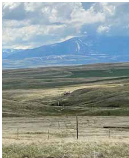
Downed poles and power lines in Geysler area. | PHOTO COURTESY OF SCOTT OLSON
