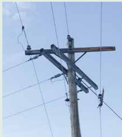
Storm damaged crossarm dangling from a power pole. | PHOTO COURTESY OF SCOTT SWEENEY
