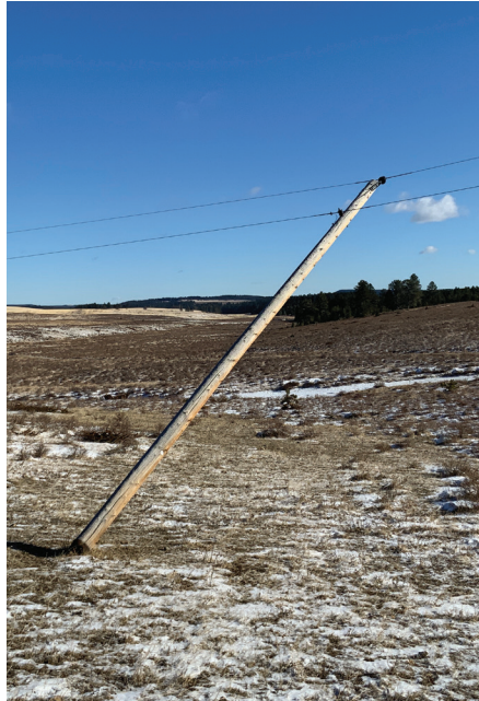
The windstorm in January broke 21 power poles and had outages affecting 1,982 Fergus Electric meters. | FERGUS ELECTRIC PHOTO
