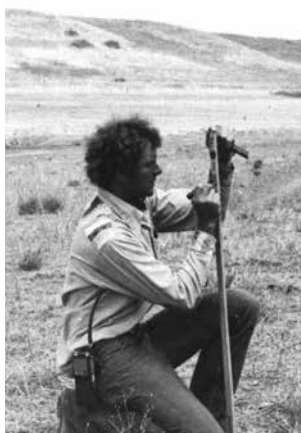
Scott Sweeney staking for new FEC building.
